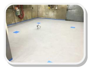
CPE installed a 1/4" thick urethane slurry system and created 2" high coving in certain rooms in the food processing area. The floor surfaces were top-coated with a 100% solids epoxy with broadcast aggregate for slip resistance.
